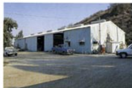
THE MAINTENANCE BARN BEHIND THE 14TH GREEN.
