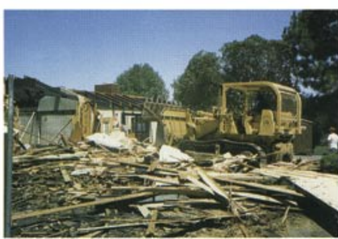
PROSHOP DEMOLITION UNDERWAY
