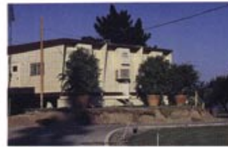
THREE MOBILE UNITS SERVED AS THE TEMPORARY PRO SHOP
