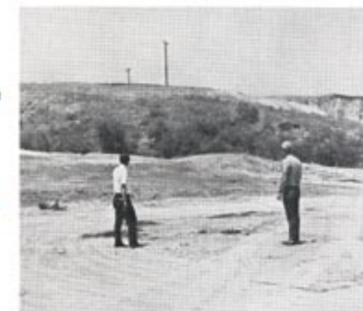
JOE DEEBLE AND OMER TINGLE INSPECT GRADING IN PROCESS
