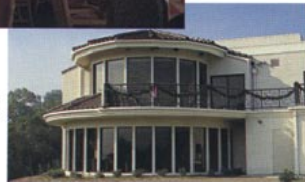
THE TERRACE ROOM IS ABOVE THE MEN'S LOUNGE
