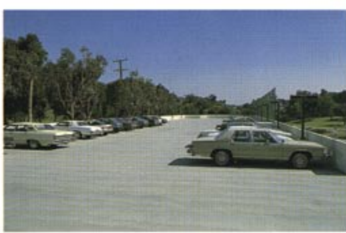
THE TWO LEVEL PARKING STRUCTURE WAS COMPLETED FIRST
